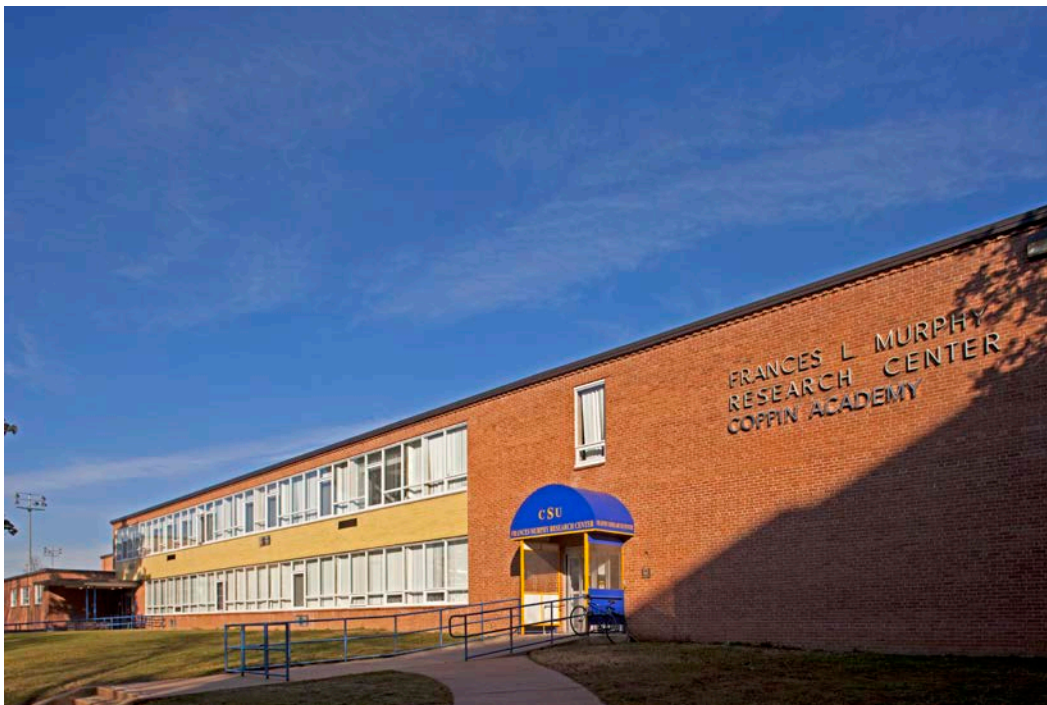
Figure 2: Frances Murphy Building - Coppin Academy
