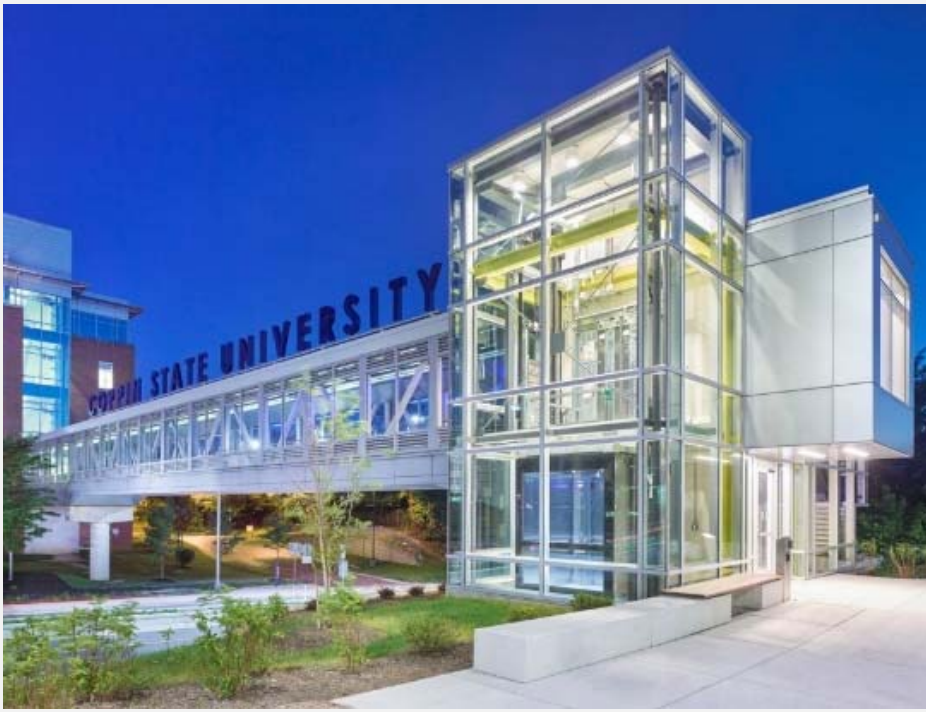
Pedestrian Bridge over W. North Ave.
